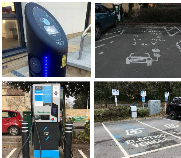
Photographs of EV charge points from field research in and around Bath
